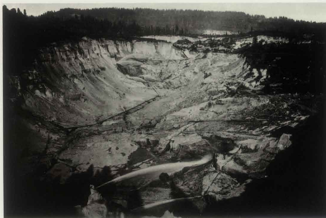
Hydraulic mining in the Sierra Nevada brought the first major man-made alterations in the natural waterscape. In the photograph at left, great streams of water under pressure are used at the Malakoff Diggings to break down walls of gold-bearing river gravel. In the photograph below, water drives a sawmill preparing timber for the construction of flumes and diversion works. The photograph at bottom left illustrates a different type of mining which became popular during the 1860s and 1870s. Here an entire river has been diverted from its course at the Golden Feather Mining Claim to provide access to the streambed. Works of this magnitude required the development of a structured work force of paid laborers. The Chinese workers seen here thus began to replace the independent miners who first opened the mountains to exploitation.
