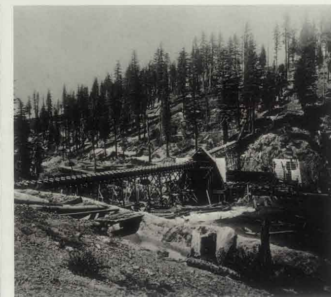
Hydraulic mining in the Sierra Nevada brought the first major man-made alterations in the natural waterscape. In the photograph at left, great streams of water under pressure are used at the Malakoff Diggings to break down walls of gold-bearing river gravel. In the photograph below, water drives a sawmill preparing timber for the construction of flumes and diversion works. The photograph at bottom left illustrates a different type of mining which became popular during the 1860s and 1870s. Here an entire river has been diverted from its course at the Golden Feather Mining Claim to provide access to the streambed. Works of this magnitude required the development of a structured work force of paid laborers. The Chinese workers seen here thus began to replace the independent miners who first opened the mountains to exploitation.
